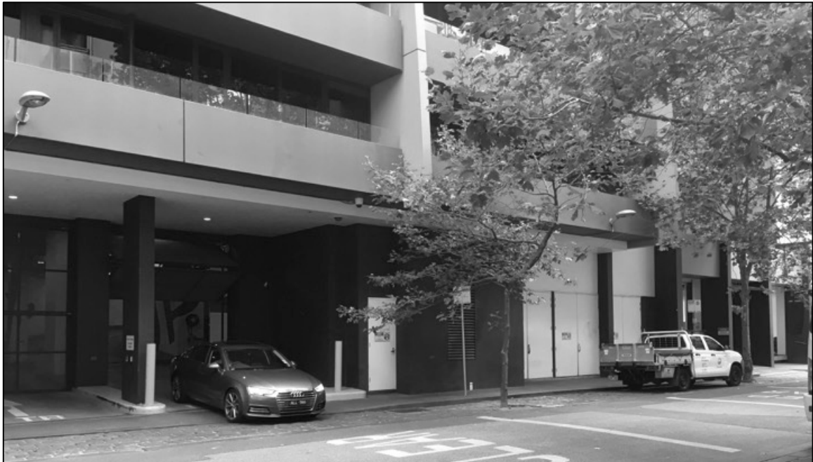
Example of poor ground floor interface
